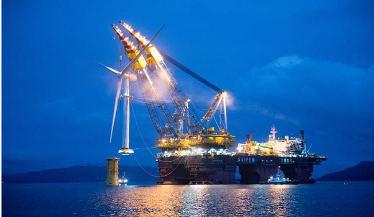
The Hywind Scotland project comprises five 6-MW Siemens Gamesa turbines. This image shows the turbines being installed on floating foundations in Stord, Norway. Courtesy: Siemens Gamesa
